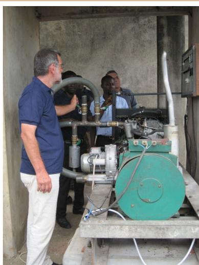
**The gasifier for off-grid electricity generation at TCC-KNUST**
