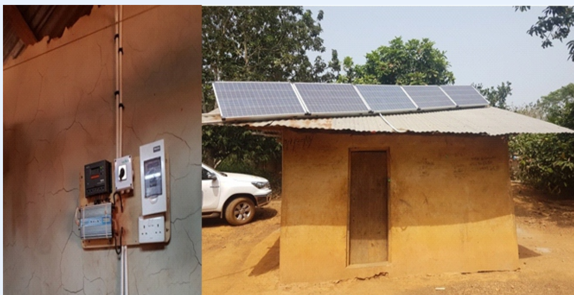
Fig 2: A solar PV installation at Agyeman, a village in Kwahu East District of the Eastern Region
