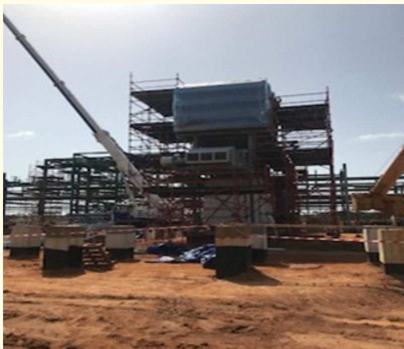
Fig 13. Installation of train 2
