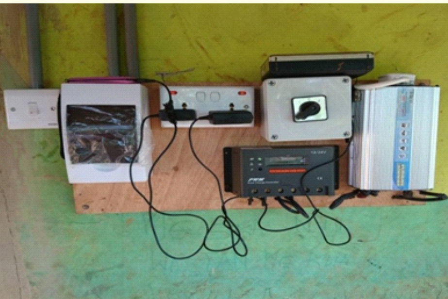
Figure 20: A system used in charging a mobile phone and radio
