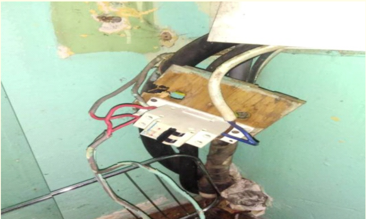
Figure 9: Sub-standard Wiring
