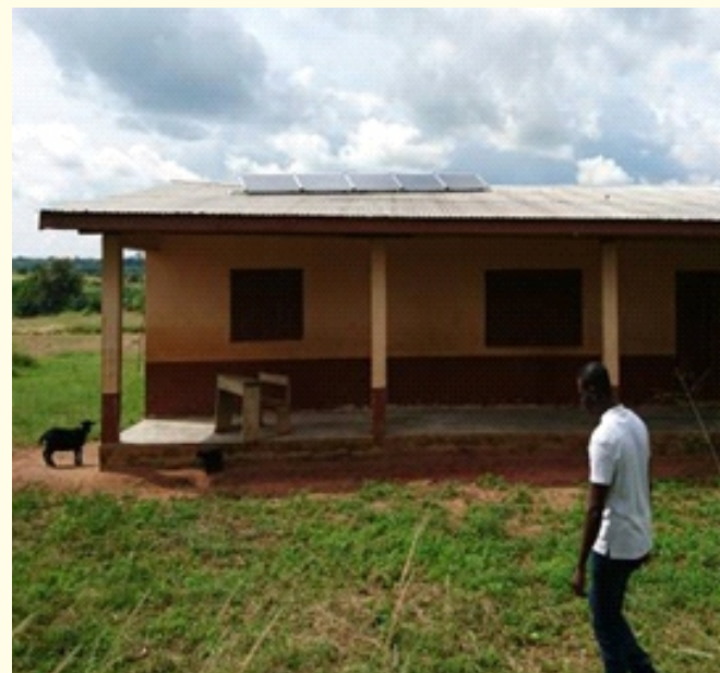
Figure 21: Solar PV System at Asesieso Basic School
