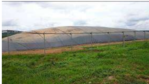
1000m 3 biogas reactor © RETT Project
