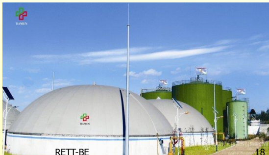
Medium and Large scale Biogas Plants (MLBPs)
