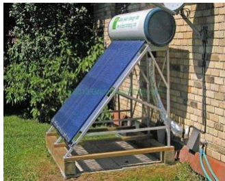
Evacuated Tubes Solar Water Heating System
