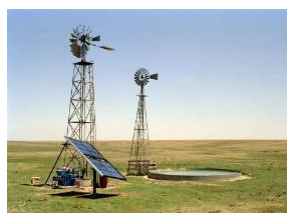
Wind/Photovoltaic Hybrid System for Irrigation
