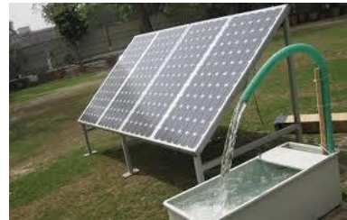
Solar Water Pumping for Domestic Use
