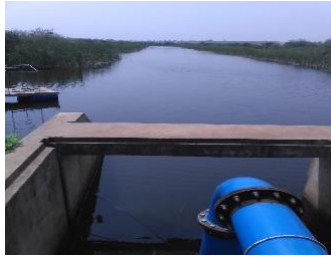
Water intake point
