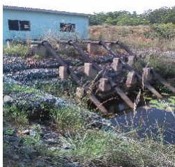
Water intake point
