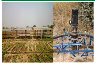
$1\,5kW$  solar PV and 30kW pump for irrigation
