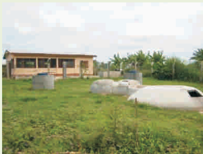
Figure 9: Initial state of the Biogas Plant at Ejura
