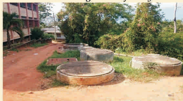
Biogas digesters with effluent storage and pump
