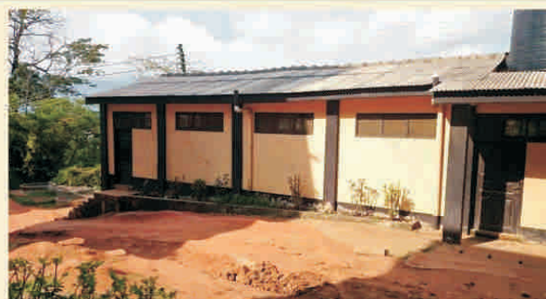
16-seater biogas toilet facility
