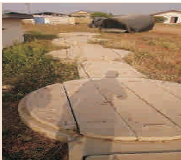
Tamale SOS biogas plant
