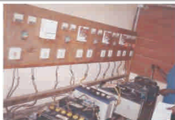
Figure 28: Initial state of the solar battery charging centre at Wechiau showing batteries being charged.
