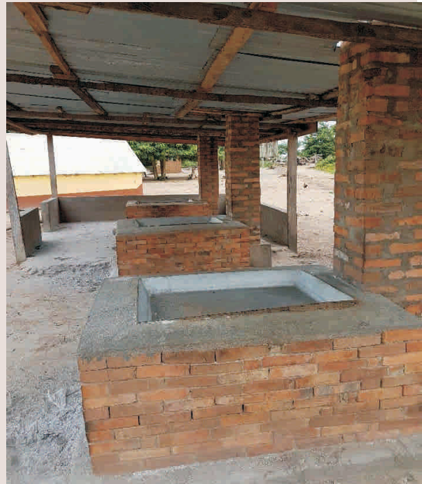
Lawrence stove installed at Adaklu in the Volta Region for gari processing
