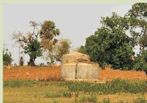
Concrete storage tanks at Tampezua for the pumped water
