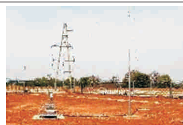
Weather station to explore the potential of CSP in the region
