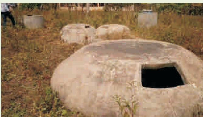
Figure 10 : Ejura Slaughterhouse Biogas Plant choked with sand and rubbish
