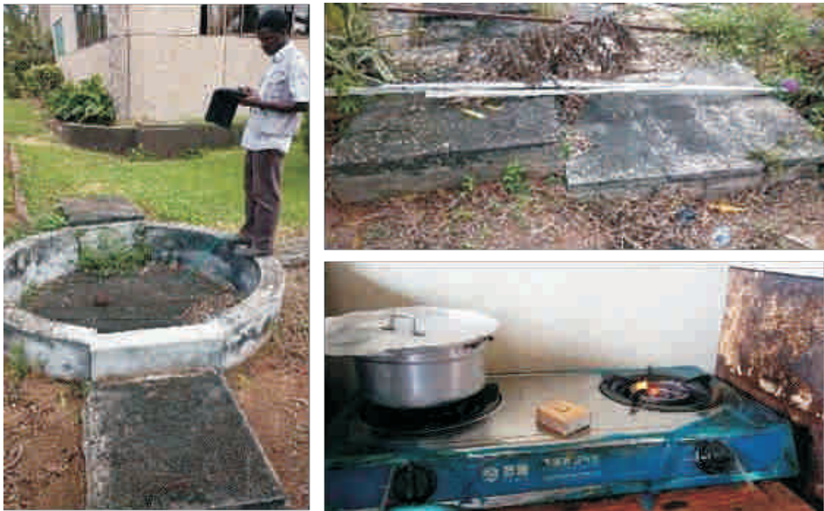
Figure 8: Biogas Plant used to supplement LPG in cooking at Ntiamoah Hotel
