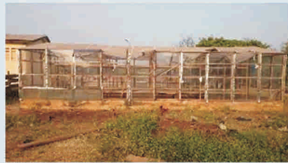
Sekyedumase solar dryer showing shuttered glass
