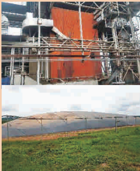
1000m 3 biogas reactor.
