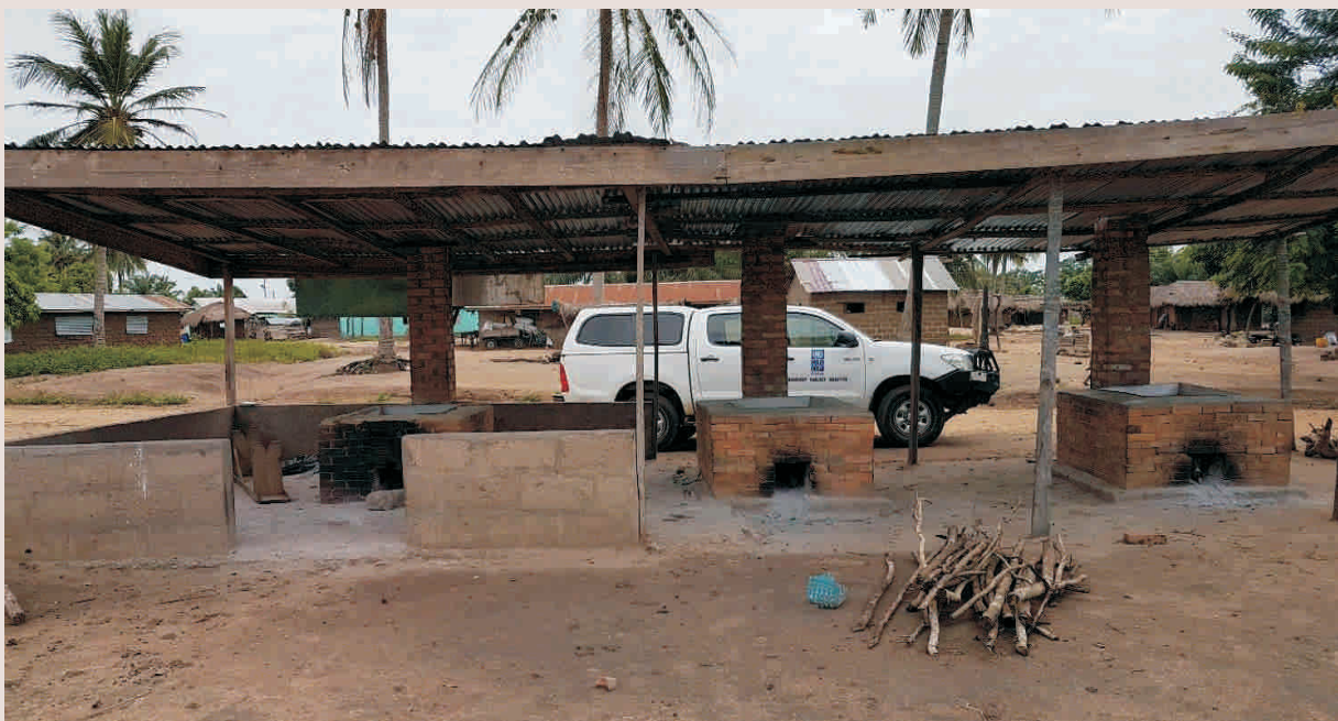
Three Lawrence Cookstoves built with burnt bricks
