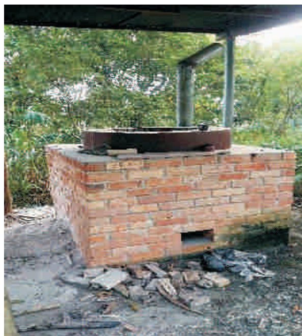
Figure 2: Institutional rocket cookstove built at TCC
