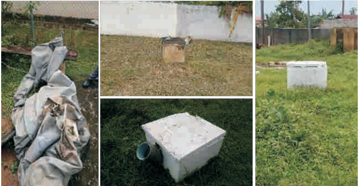
Figure 5: Abandoned Biogas Plant at Koforidua Hospital
