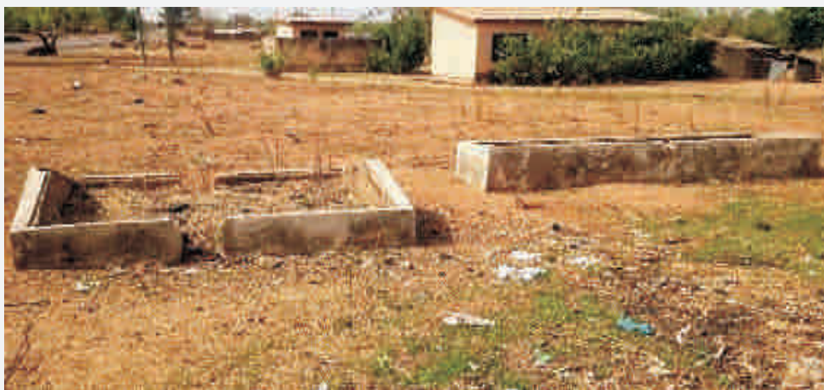
The deplorable state of the water stills
