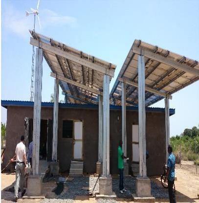
Solar PV Panels mounted on high structures and distribution lines
