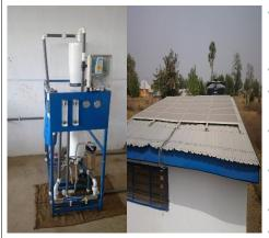
Panels on the roof powering water filtration system
