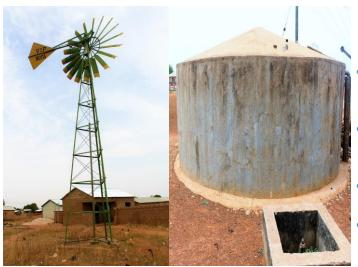
Poldaw windpump and storage tank provided for irrigation
