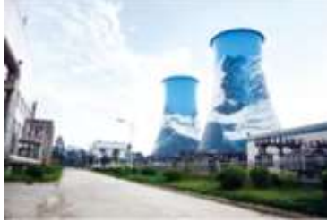
Chengdu Sanwayao Thermal Power Co., Ltd.
