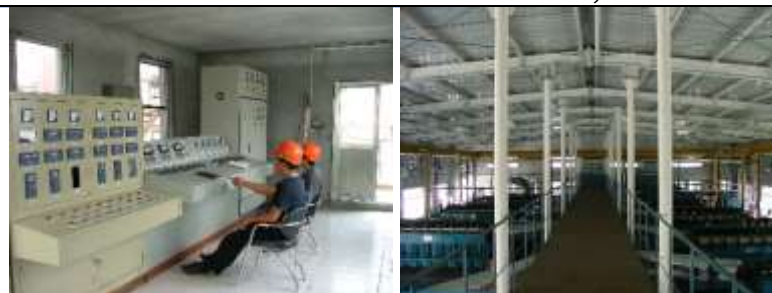
b. control room
