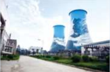
Chengdu Sanwayao Thermal Power Co., Ltd.
