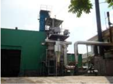
d. steam boiler
