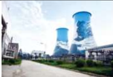
Chengdu Sanwayao Thermal Power Co., Ltd.
