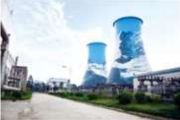
Chengdu Sanwayao Thermal Power Co., Ltd.
