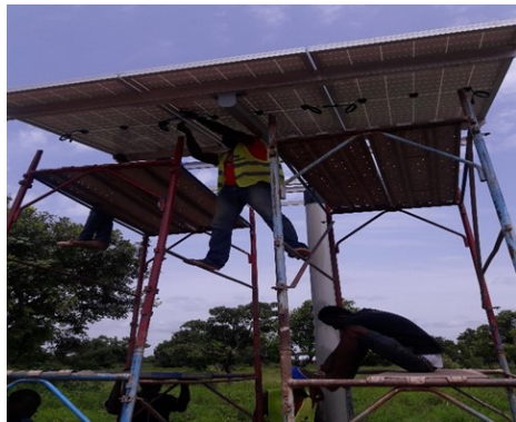
Panel Installation (Photo credit: Power World Ltd.)
