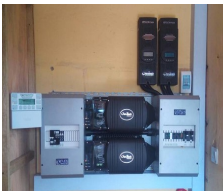
Complete Outback Inverter and Charge Controller (Photo credit: Power World Ltd.)
