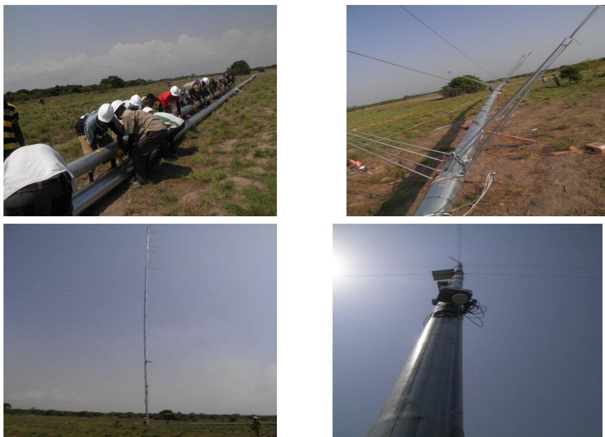
Figure 2: Installation of Wind Measuring Mast at Gomoa Fetteh
