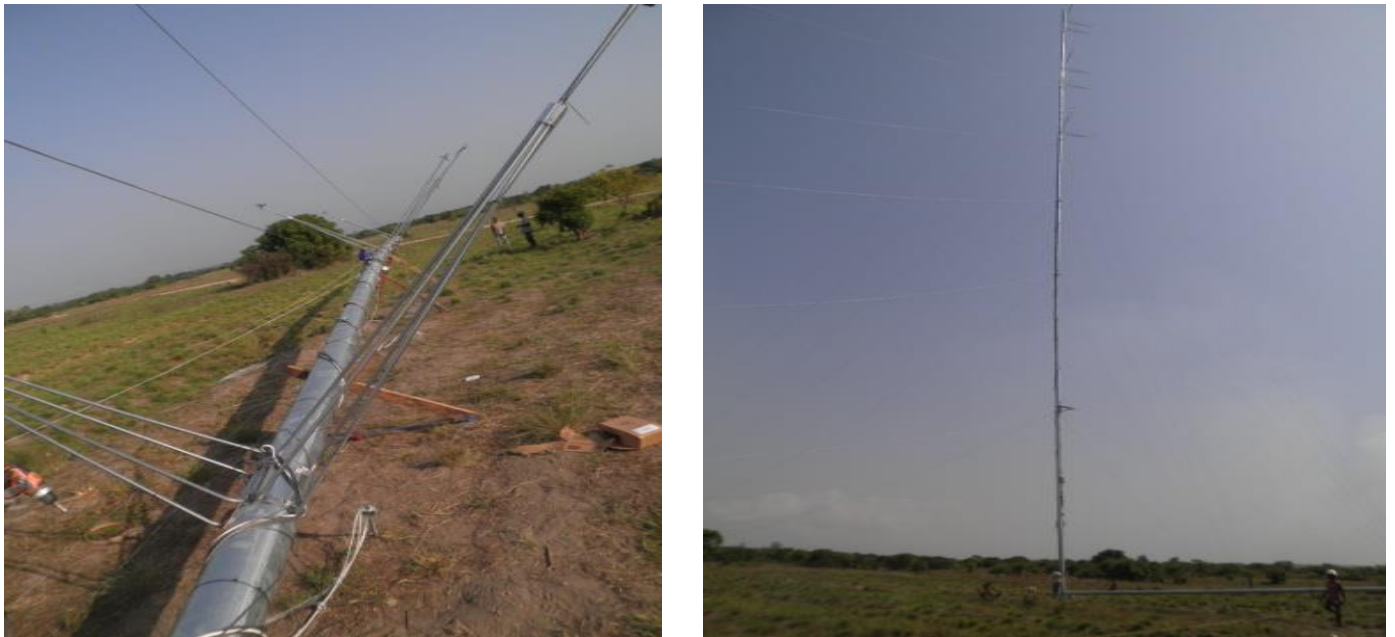
Fig. 5: Installation of wind measuring equipment at Sege in the Greater Accra Region
