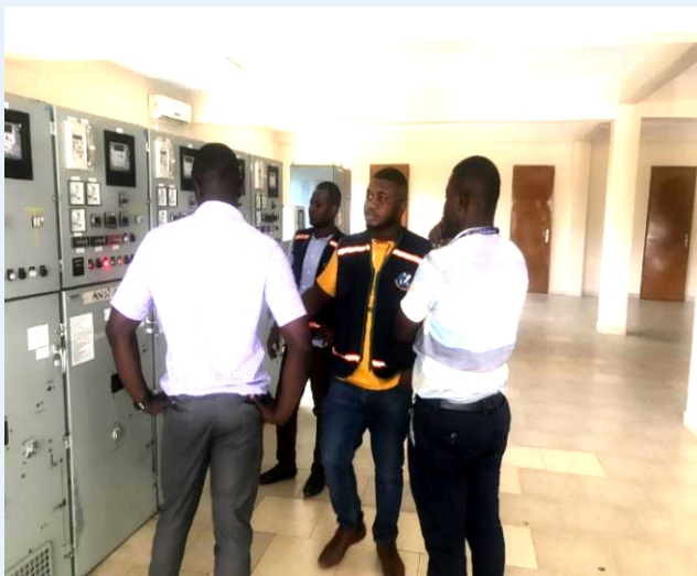
Fig 3: Inspection of Circuit Breakers in a Primary Substation
