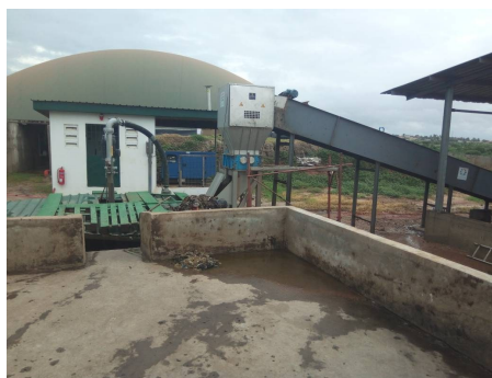
The Safi Sana waste-to-energy plant (Photo credit: Lovans Owusu-Takyi)
