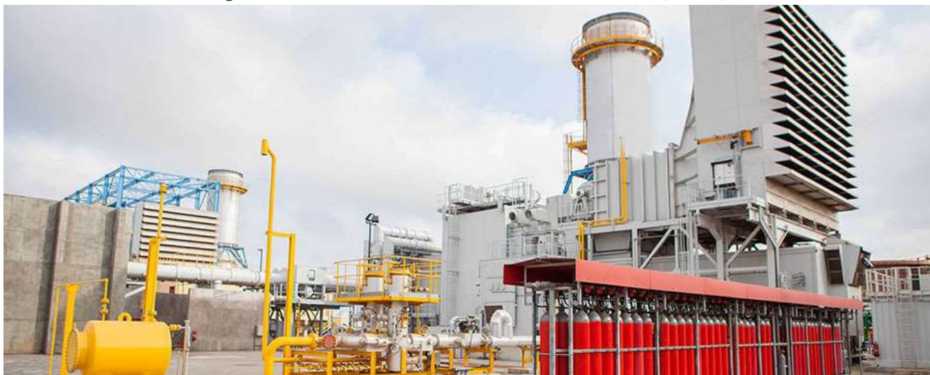
Figure 1: A view of the Tema CENIT Thermal Power Plant (TCTPP)
