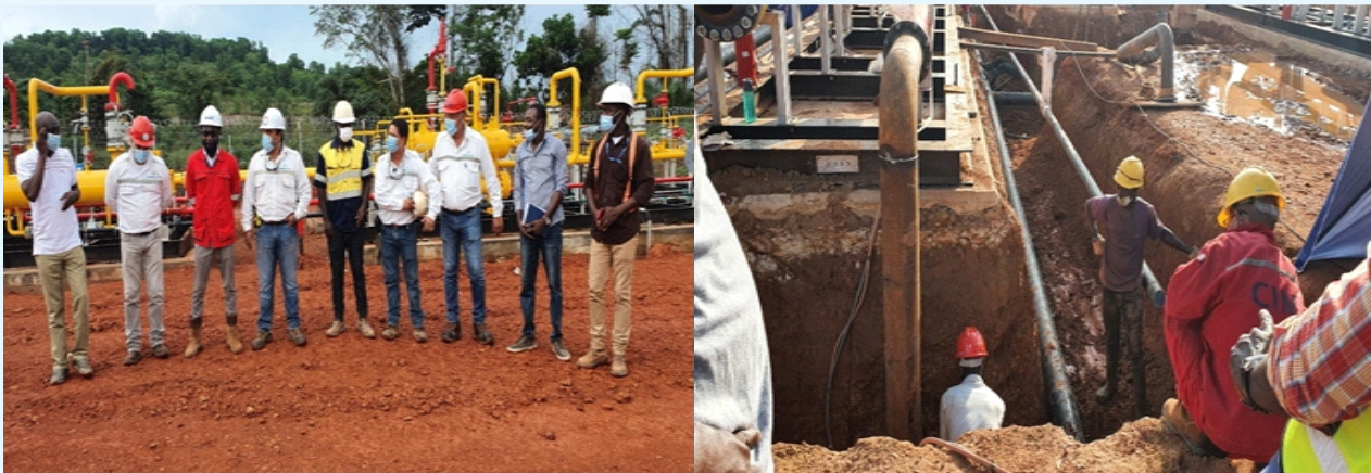
Fig. 3 Engagement of some local artisans in welding by Inspection team of the Commission.
